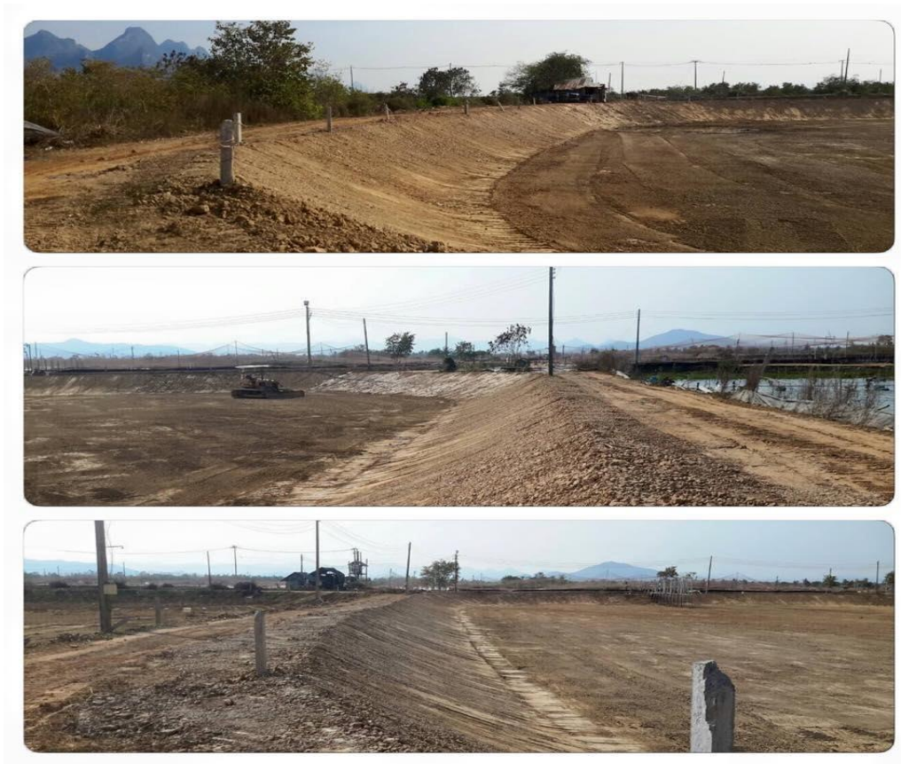
Fig 1: Preparation of pond bottom
